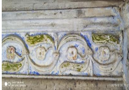
Figure 10: Frieze design on the parapet
