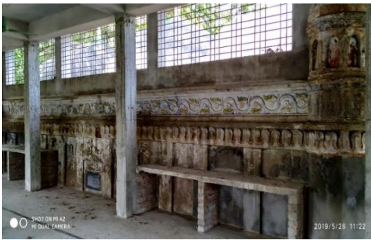
Figure 11. Merlon and frieze design on the parapet
