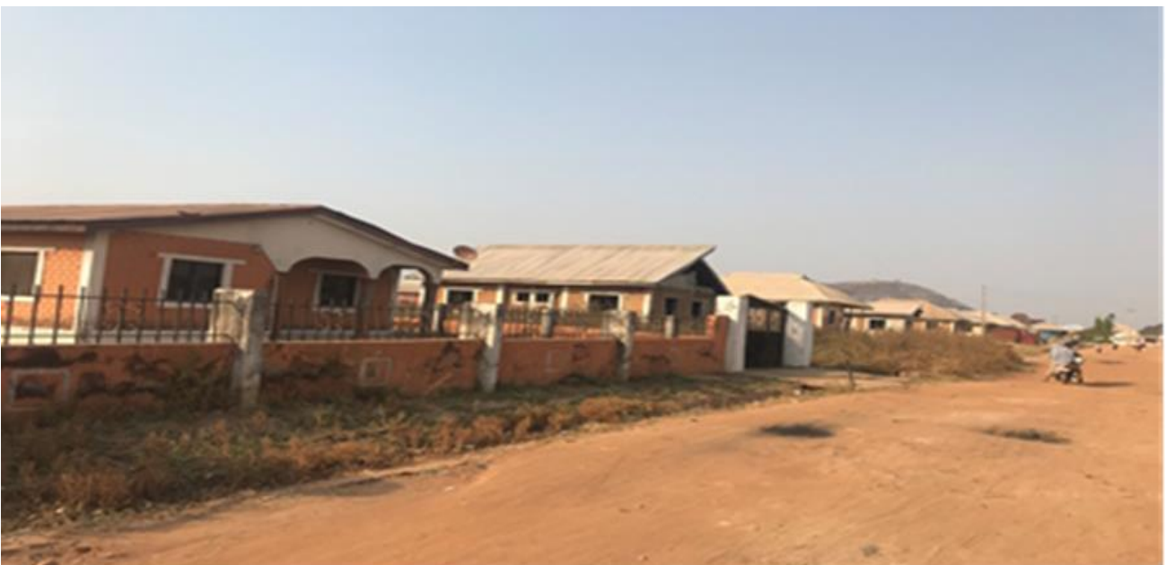
Plate 2: Road and drainage state of maintenance in Royal valley housing estate
