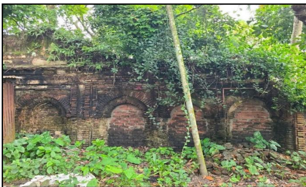
Image 5: Present boundary wall of Sreepur Zamindar house
