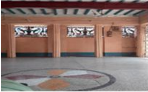
Figure 11: Interior view of the South-east Section of the temple, where some Indo-European columns and Iron beams were used in the Roof (Photograph by authors, taken during field study, January 2026)
