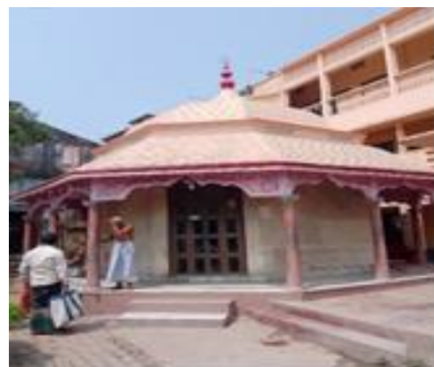
Figure 7: Exterior, In view of the octagonal building showing columns and spire detail (Photograph by authors, taken during field study, January 2026)
