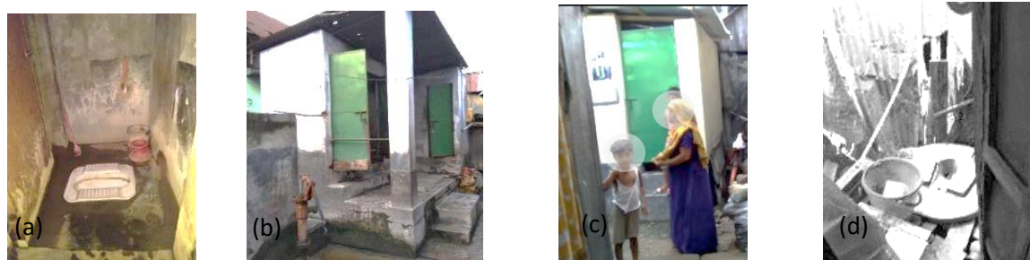
Figure 3. Sample toilets (a) Single HH, Single pit; (b) Shared HH, Septic tank; (c) Shared HH, single pit; (d) Single HH, Hanging Toilet (source: author).
