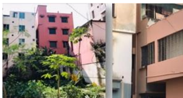
Figure 9. Violation of setback rule.
