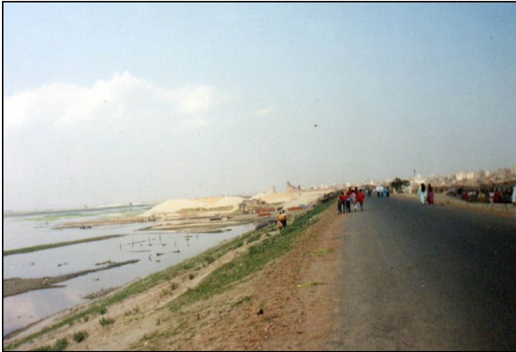
Fig. 16. The flood protection embankment of Dhaka, an emerging open space.
