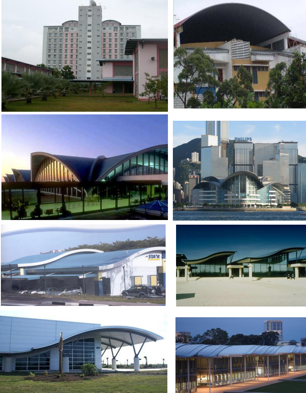
Figure 1. Parabolic and doubly curve thin shell profiled steel sheet roofing.
