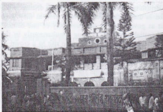
Fig.- 2.e. Nagar Bhaban (Demolished in 2003)
