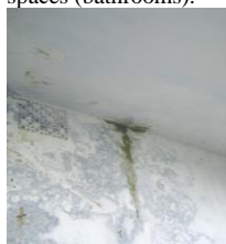
Fig. 9. Effects of horizontal dampness water is coming through the sidewalls laterally
