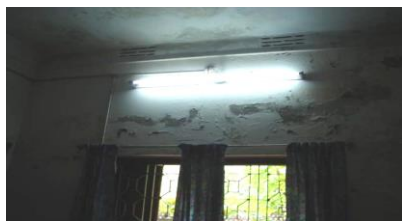
Fig. 8. Effects of horizontal dampness
