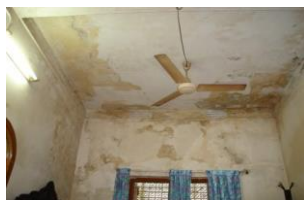
Fig. 10. Presence of falling dampness coming.
