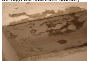
Fig. 11. Presence of falling dampness, where water is through the cracks or voids of slabs.
