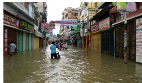
Figure 13. Flood in Maldapatti, 2017.
